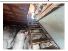
1. Hand railing was not provided to the 01 staircase leading from first floor towards ground floor (shed 2)
