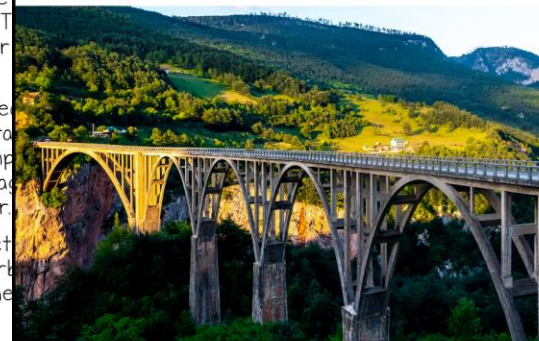
Similar structures can have different forms (e.g., not all bridges are arches).
