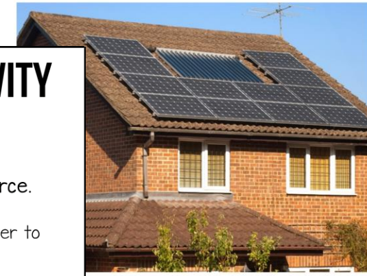
of Solar Panels on the Roof of a House
