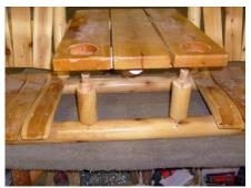
4. Position 9" spindles and insert tenons into pre-drilled holes in seat bottom. Rotate table down and insert upper spindle tenons into pre-drilled holes in table underlay. Use 2" screws to capture all tenons in table underlay and seat bottom as shown. *Note: When rotating table into position, be sure table brace from Step 3 rests on top of seat bottom horizontal log (see step 5 for visual).*
