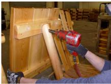
3. Position angled end of table brace to bottom of tabletop underlay, center and secure brace with a 2 ½" lag bolt and washer as shown.
