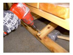
5. Use 3 3/8" lag bolt with 1/4" washer to secure angle brace.
