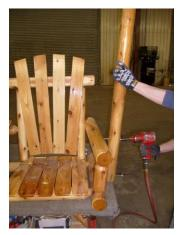
8. Attach swing hangers to arm assemblies using 5" lag bolts and 5/16" washers. Align pre-drilled holes on swing hanger with pre-dimpled marks on swing arm assemblies (both upper and lower arms).
