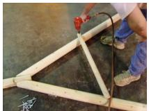
10. From machine bolt, measure 32" down each swing leg. At this location, secure 35" horizontal brace using 4" lag bolts and 1/4" washers.
