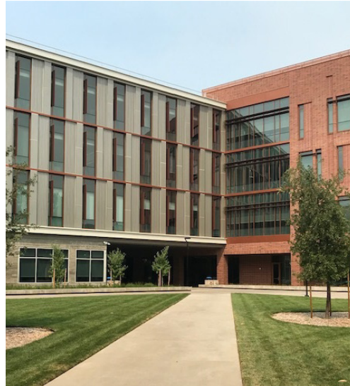
The new Geoscience Building
