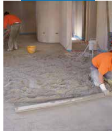
Spreading the mix with Mapescreed 704 admix
