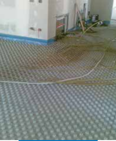
Preparation of the heating/cooling system
