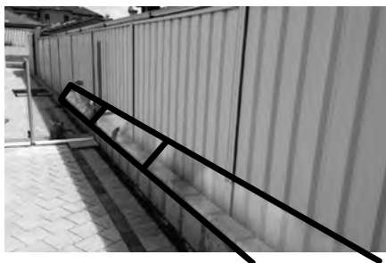
Oscillot® installation with rigid polycarbonate blocking off ledge on raised retaining wall eliminating it as a potential platform.
