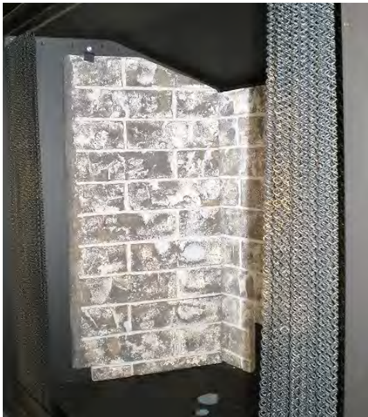
Step Three: Tilt and slide left and right Side Liners into place.
