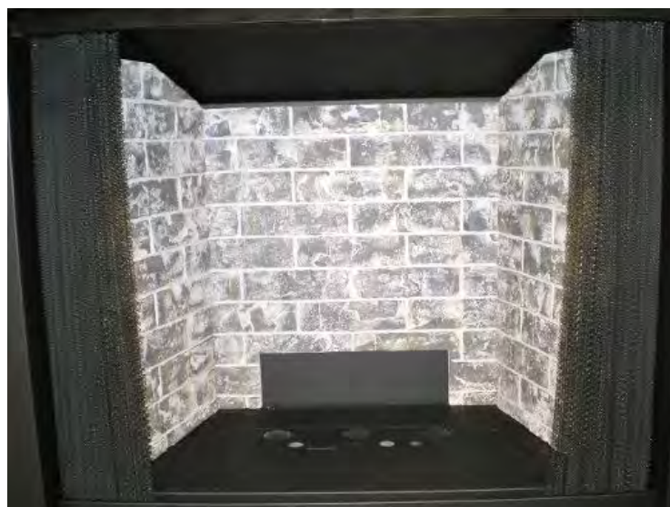
Step Three: Tilt and slide left and right Side Liners into place.
