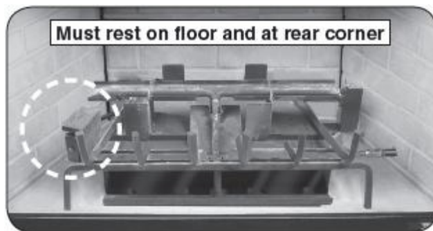
Fig. 13-1 Place heat shield
