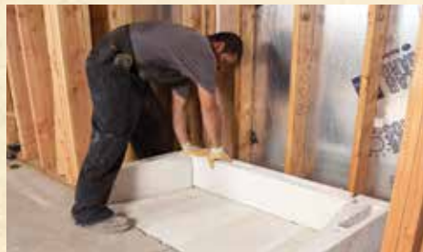
1. Installing base and first course
