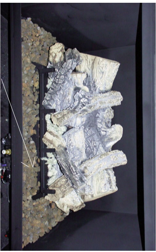
Step (10) Place crushed rocks onto firebox bottom. (NOTE: Do not place crushed rock onto burner tubes)
