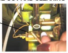
Gently pull out the propane feed and wipe off the tip where the propane is released. If there is a lot of black coming out just tap on the side of the pilot tube with a screw driver to get all the buildup out. Put everything back together and start your heater. This should be done once a month for assuring a long life of your heater.
