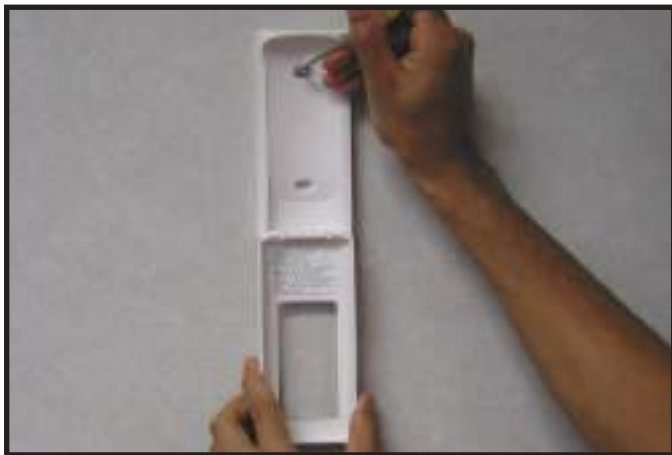
Figure 11.2. Mounting Remote Control Housing
