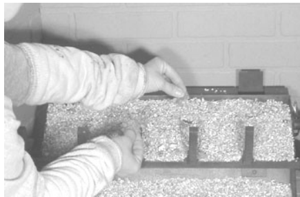
Figure 4c-Placing remaining rock wool
