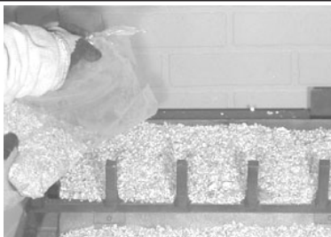
Figure 3 Placing Vermiculite
