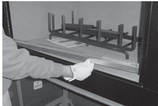
Figure 1 - Install the Door Track
