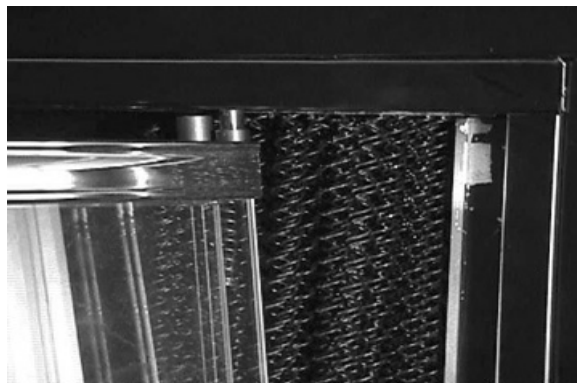
Figure 7 - Pivot Pins/Top Door Track
