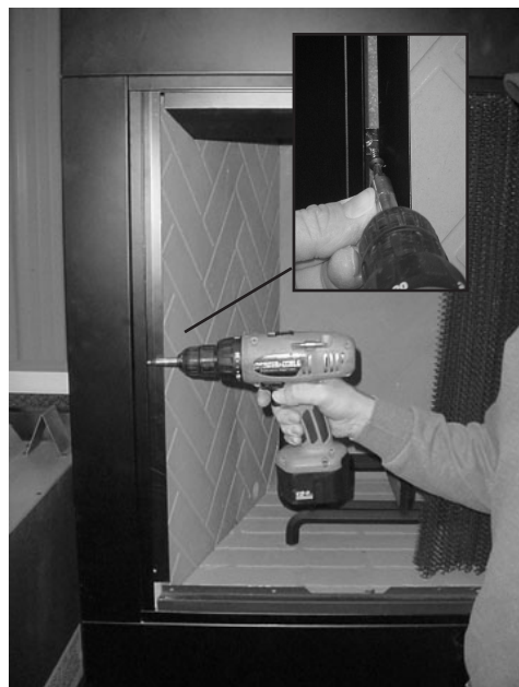
Figure 5 - Fastening the Side Filler
