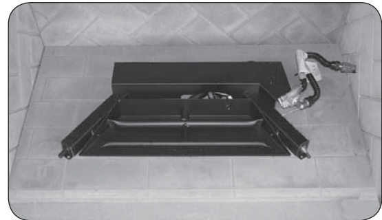
Fig. 16-2 Center burner in fireplace
