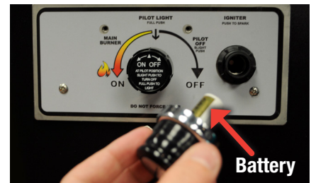
Figure 10.6 – Slide battery into spark igniter unit.
