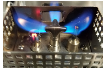
Figure 10.2 – Pilot flame coverage of thermocouple.
