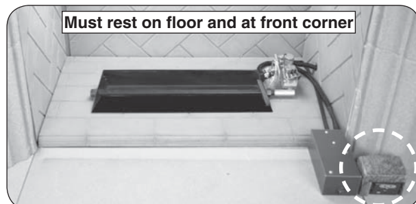
Fig. 9-3 Place decorative heat shield
