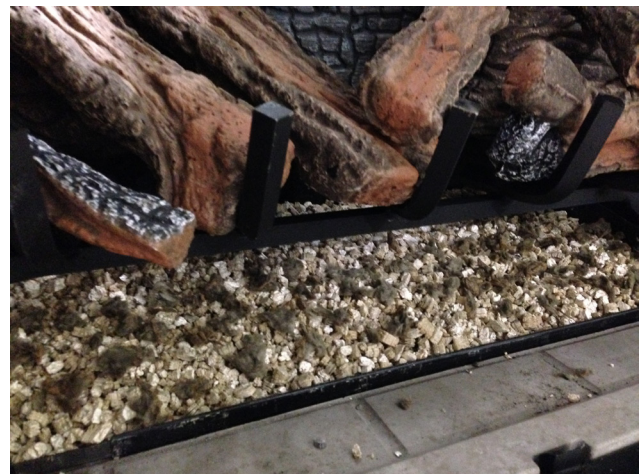
Figure 22 - Completed Installation of Vermiculite and Embers
