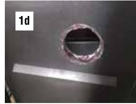
1d. Seal the exposed insulation with Foil tape.
