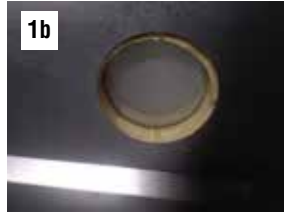
1b. Remove 5" round piece of Insulation.
