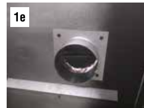
1e. Attach the collar and plate with 4 sheetmetal screws. In some instances there may not be pre-drilled capture holes.
