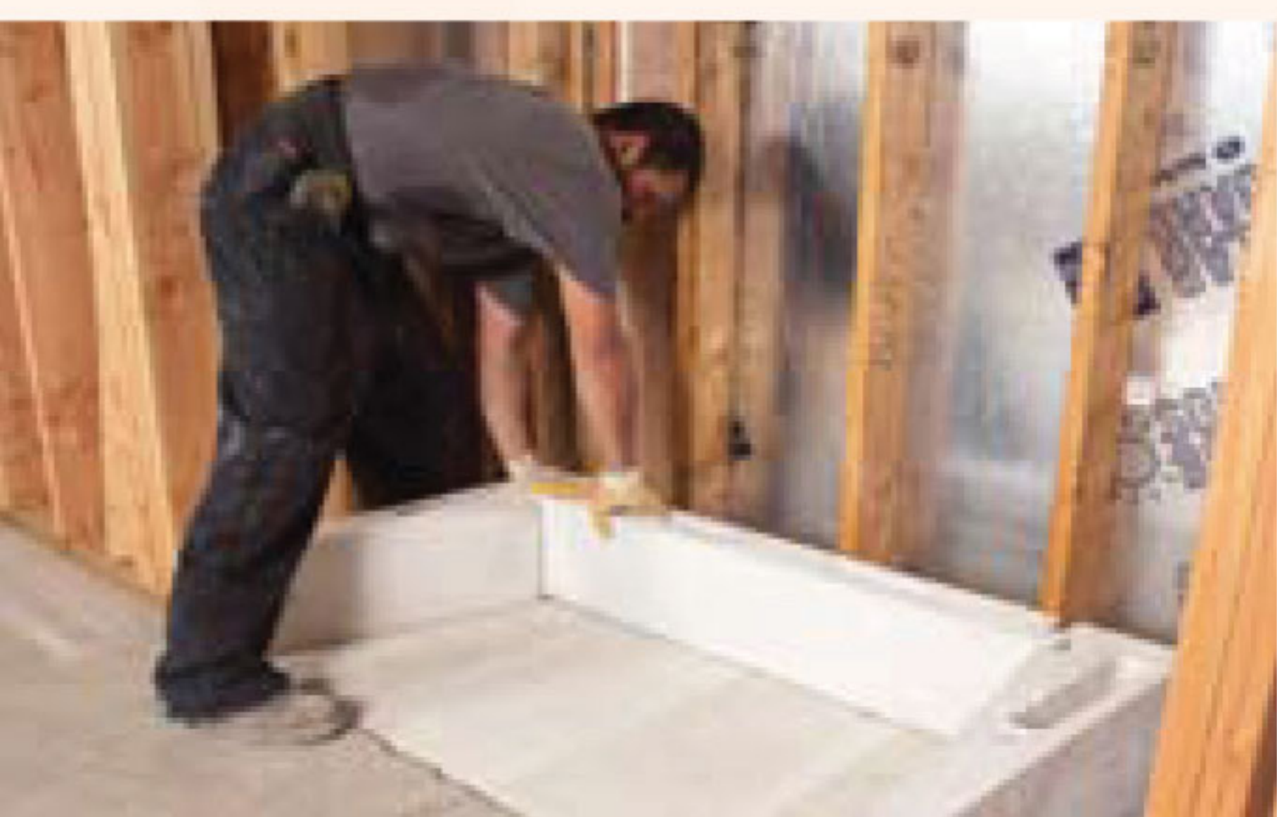
1. Installing base and first course
