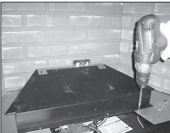
Figure 14.28 Remove Screws Attaching Front Burner Support
