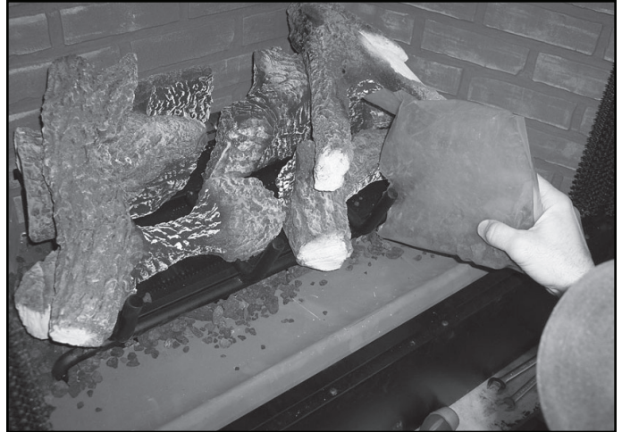
Figure 14.21 Placement of Lava Rock
