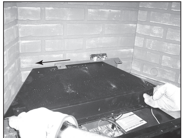
Figure 14.30 Side Burner Assembly to Left
