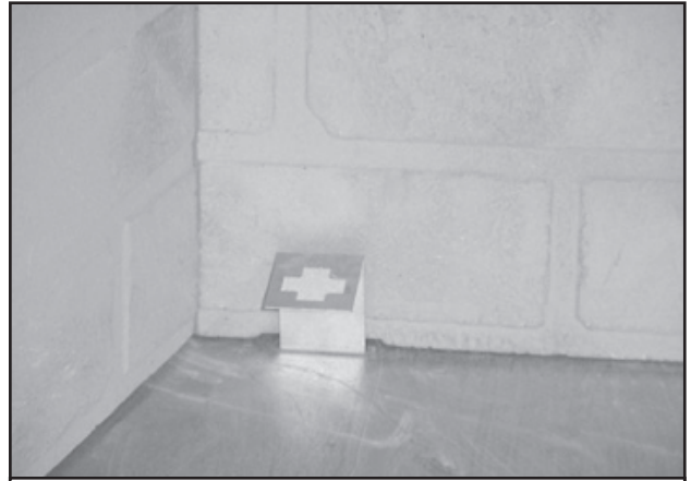
Figure 8.8 Grate Retaining Bracket in Place
