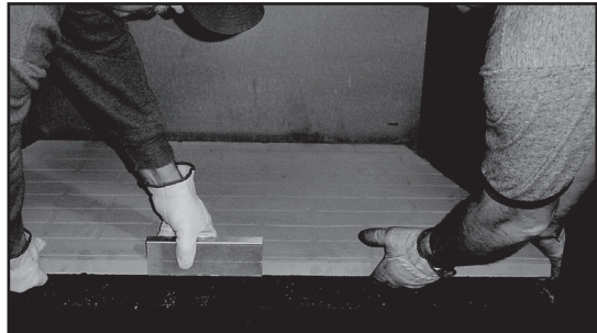
Figure 3.10 Lifting Out Hearth Stone
