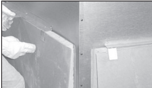
Figure 3.6 Unpack Back Refractory
