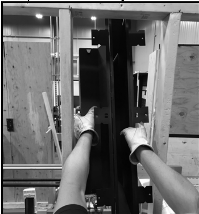
Figure 5.15 Turn Plenum Vertically to Clear Framing Studs
