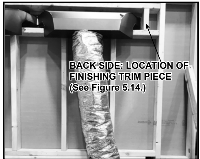
Figure 5.29 Flex Vent Installed with No Kinks
