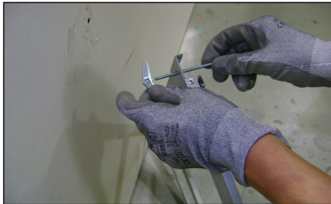
Figure 4.10 Toggle Bolt Installation through Mounting Bracket
