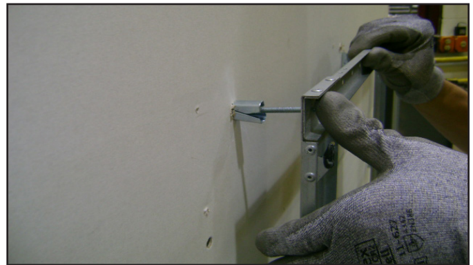
Figure 3 Installing Anchors in Hollow Wall
