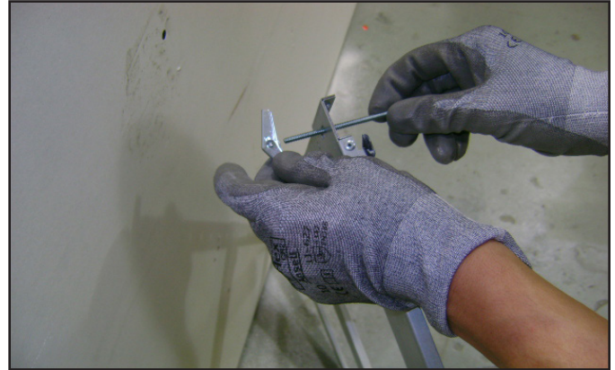
Figure 2 Toggle Bolt Installation through Mounting Bracket
