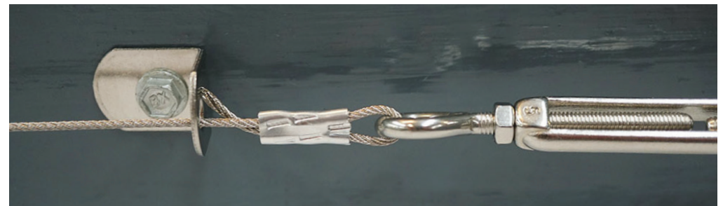
Guide wire fed through eyelets to create a wire framework for attachment to netting.
