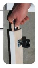
Slot the end of the side rails into the end rail, inserting the dowells and bolt to the pre-drilled holes.
