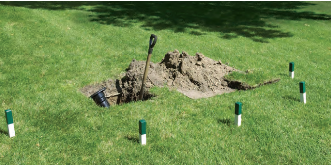
Mark off repair areas.
