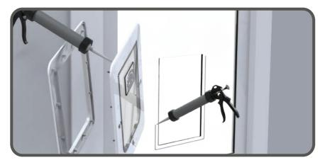
Refer to Steps 1 and 2 of "Installation". Place a bead of construction silicon around the internal section of the pet door and on the surface around the cut out to provide a weather seal. Tunnel is not required.
