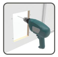
Insert outer frame into opening and mark screw holes. Drill each of the screw holes using a 8mm (5/16") drill bit.
