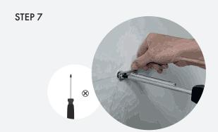
Place the concealed shelf supports over the fixings and screw lightly in place using the M6 bolts provided.
