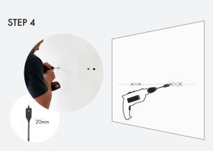
Using a 20mm spade bit, drill a hole on each of the outer marking to accommodate the Gripit fixings.
