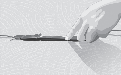
Fig. 2. Groove for joint of cold and heating cable
