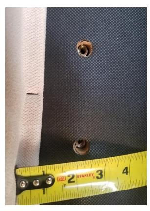
3. Cut fabric to expose the holes. Once holes are exposed, you are now ready to place the rail bracket to the bed.
