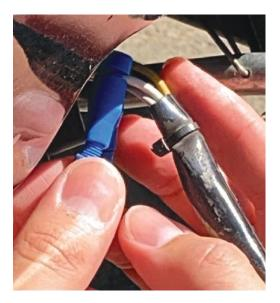
Tighten the small end of the Posi-Tap connector snugly which presses and holds the exposed wire end to the binding post creating a secure electrical connection.
