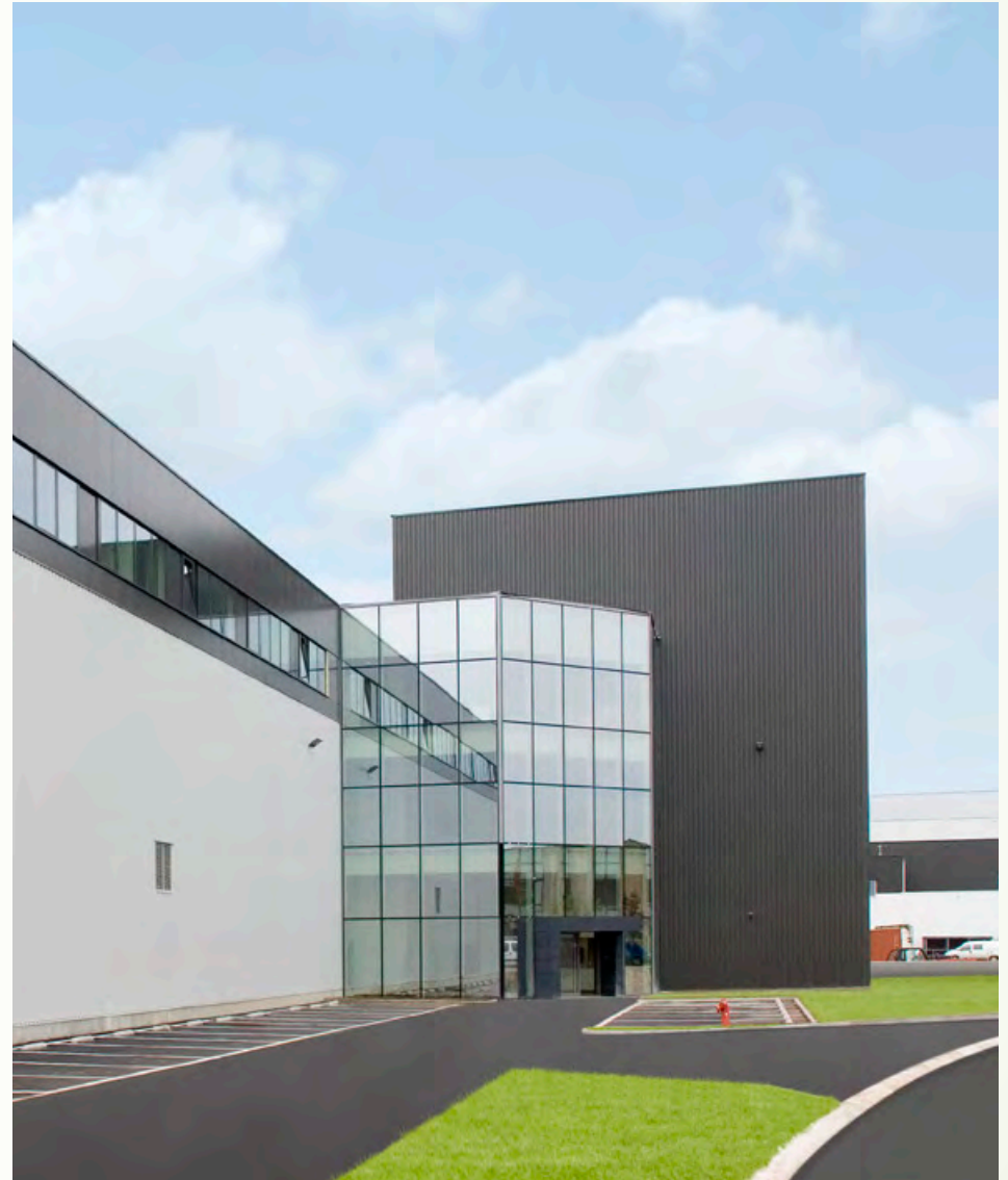
Manufacturing Facility, Aalst, Belgium
