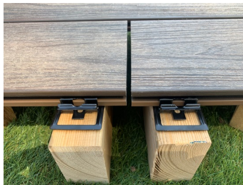
Double joist under butt joints
