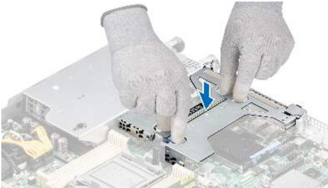
Figure 63. Installing the Riser 2c
