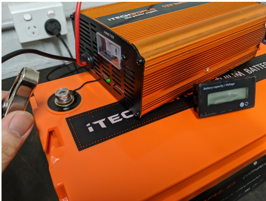
Temporarily removing the negative charger clamp
