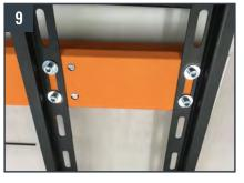
Position the TV bracket and insert the 4 bolts with washers.
