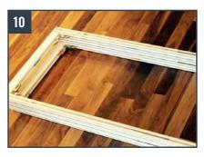
It it important that the colored labels on the small profiles are aligned with the colors on the large profiles.
