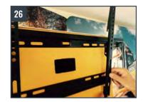
Once the rods are screwed into your TV, install the rods into the frame like SO.
