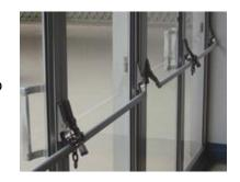
Keys cannot be used at all, including keys hung near the door, or keys available in a break-glass type container. Doors must not have a key-type lock fitted, but can have a snib lock or a 'free handle' – a door handle which is locked from the outside, but allows the handle to be opened always from the inside. Doors should be able to be opened with one hand, in a normal manner and the lock mechanism should be able to be reached by a person of any height.
