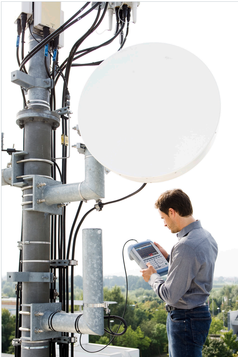
The R&S®FSH in operation during installation and maintenance of transmitter stations
