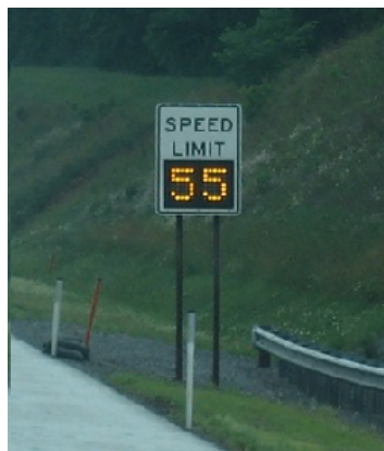
Variable Speed Limit Sign (image courtesy of: safety.fhwa.dot.gov )
