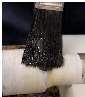
Figure 6: Applying Reinforcement resin to pipe
