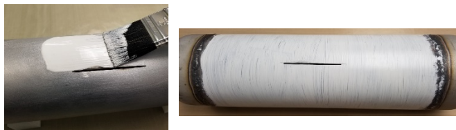
Figure 2: Applying primer to a section of pipe.
