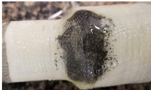
Figure 8: Fully resin soaked fiberglass application
