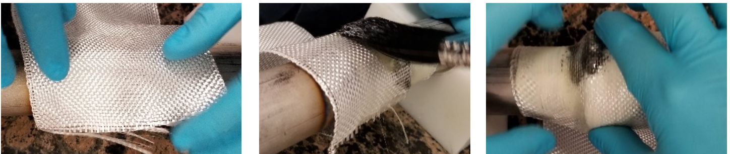
Figure 7: Applying fiberglass reinforcement to repaired area
