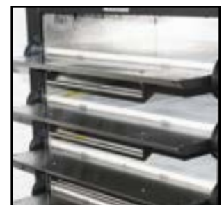
Adjustable Dampers at each deck
