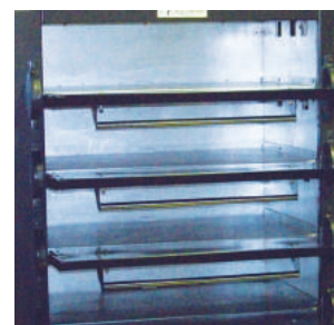
Adjustable Dampers at each deck
