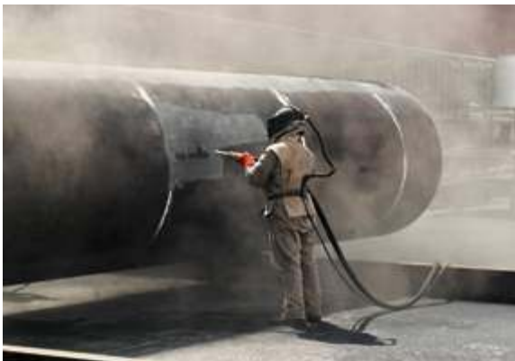
Conventional grit blasting
