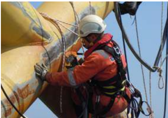
Bristle Blaster® on an offshore platform
