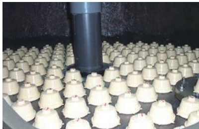
Nozzle Plate underdrain system
