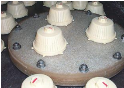
Internal Nozzle Plate Service Hatch
