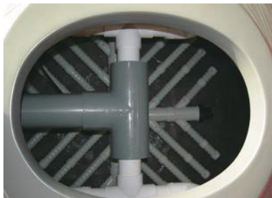
Lateral underdrain system
