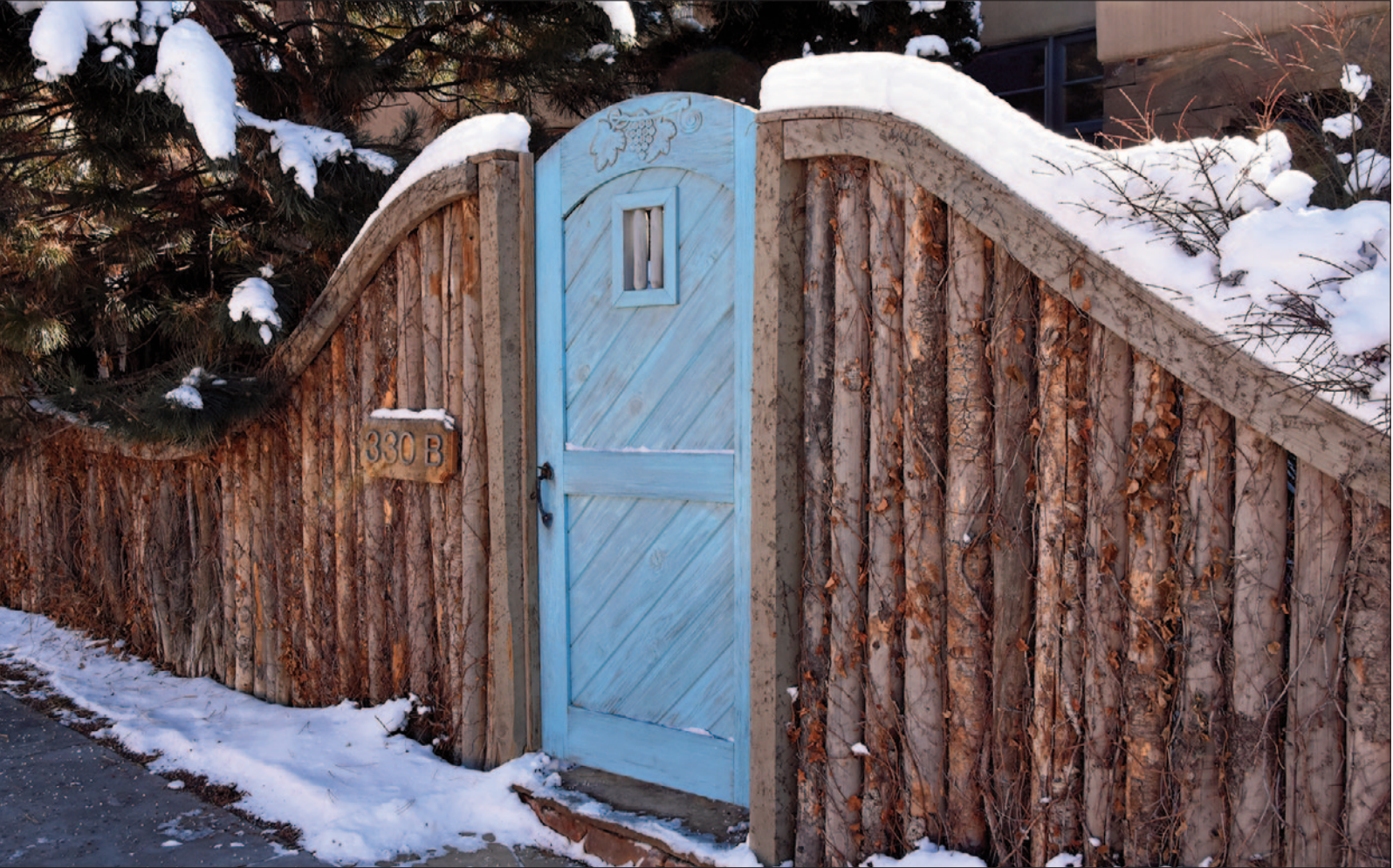
Wall built out of logs in Santa Fe style.
