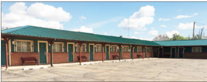
The motel is located just a few blocks east of the iconic U-Drop Inn Café and Tower Conoco Station.
